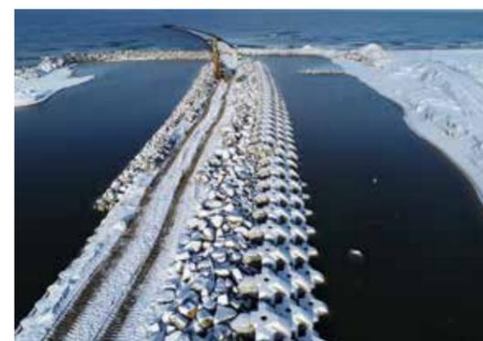
The channel stretches over 1.5 kilometres with a width varying from 25 to 120 metres. It is equipped with 61-metre long and 17-metre large rotating bridges, while the associated buildings will cover an area of 1,090 m<sup>2</sup>. Located outside the spit in the Gdańsk Bay, the two breakwaters have respective lengths of 900 and 300 metres and form a protective harbour.
