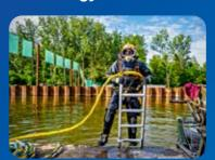
The project uses underwater concrete to minimise disturbance for the environment and to reduce to automatically generate drawings. and concreting of the floor are TWIN-16, which includes the carried out underwater. Then, the water is pumped out to create a dry construction pit in which the rest is built. Less concrete is required, thus reducing CO<sub>2</sub> emissions.
