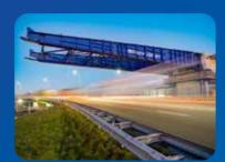
This imposing blue steel structure is the launching nose of the flyover. It was installed at the front of the first segment to balance out the weight equally and covers the distance between the different piers. In addition, it limits the internal stresses as the structure cantilevers over the existing infrastructure,
