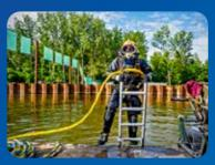
The project uses underwater concrete to minimise disturbance for the environment and to reduce to automatically generate drawings. and concreting of the floor are TWIN-16, which includes the carried out underwater. Then, the water is pumped out to create a dry construction pit in which the rest is built. Less concrete is required, thus reducing CO<sub>2</sub> emissions.
