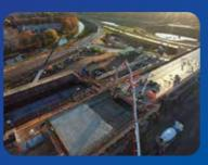
A temporary production line was set up behind the northern abutment. There. each segment – about 30 metres long - is cast in relation to the previous one and gradually pulled over the Terbreaseplein, until the whole structure reaches the southern abutment. This happens at a low pace, i.e. 4 m/h, and cannot be observed by the vehicles driving ensuring a safe operation. under the viaduct.
