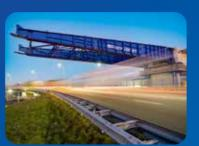
This imposing blue steel structure is the launching nose of the flyover. It was installed at the front of the first segment to balance out the weight equally and covers the distance between the different piers. In addition, it limits the internal stresses as the structure cantilevers over the existing infrastructure,
