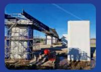
One of the engineering masterpieces is the viaduct across the Terbregseplein that passes over a railway line and motorway interchange. As closing these busy traffic lines was out of question, the consortium opted for the Incremental Launching Method, which includes gradually pulling the structure across the Terbregseplein, enabling traffic at
