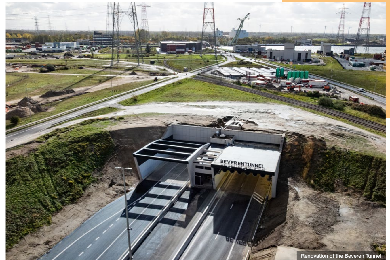
Renovation of the Beveren Tunnel
