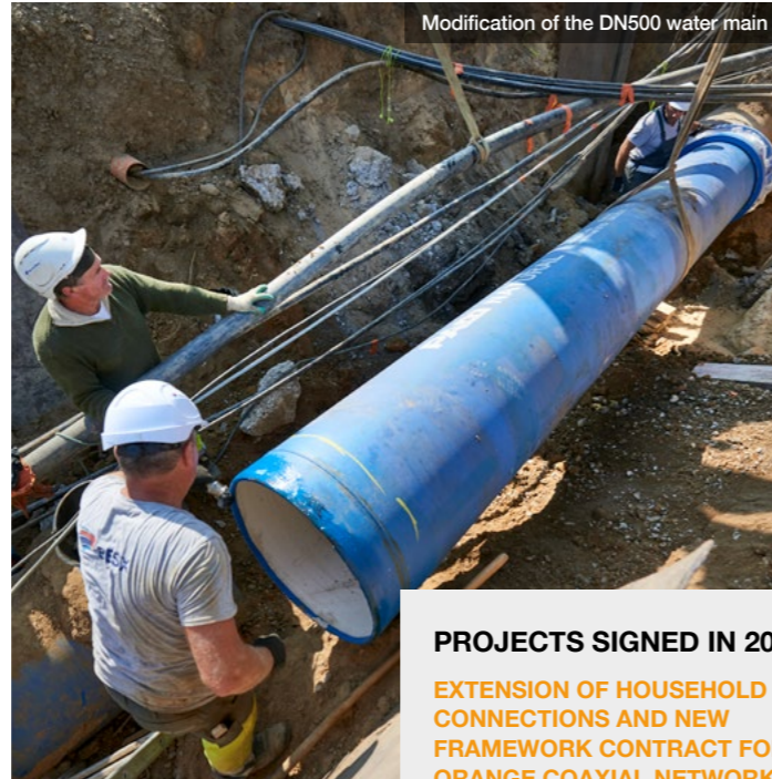
Modification of the DN500 water main
