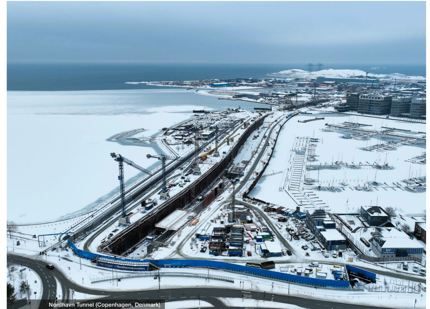
Nordhavn Tunnel (Copenhagen, Denmark)
