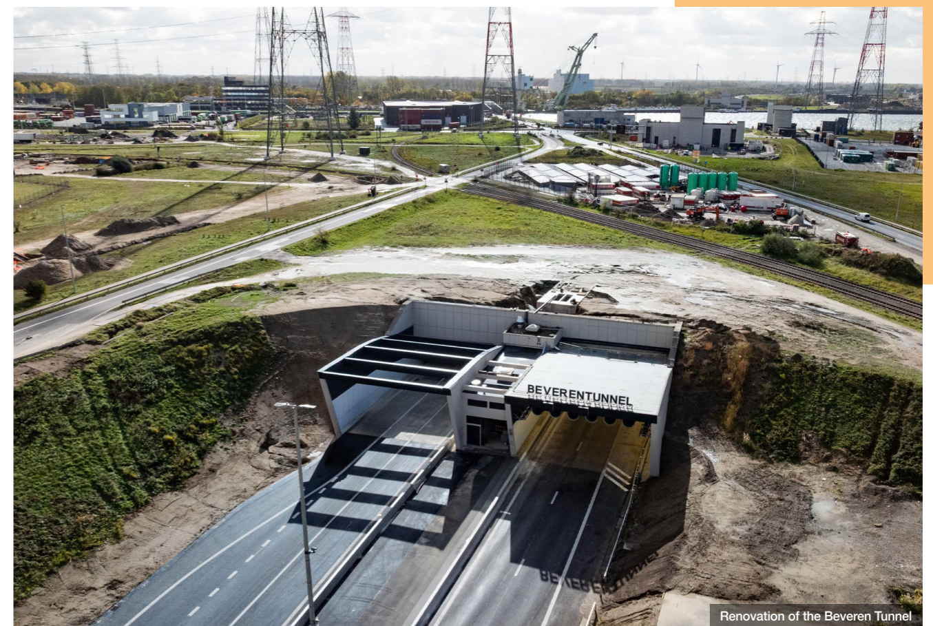
Renovation of the Beveren Tunnel
