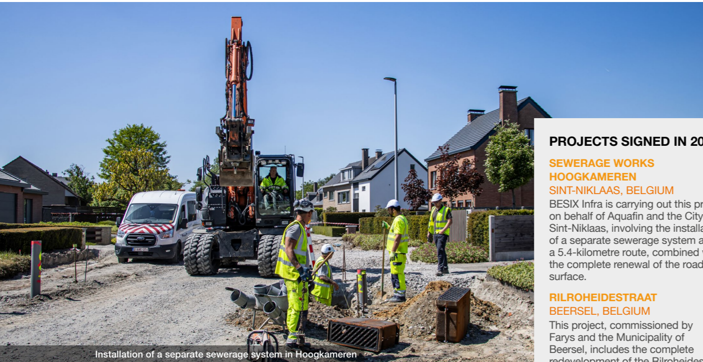
Installation of a separate sewerage system in Hoogkameren
